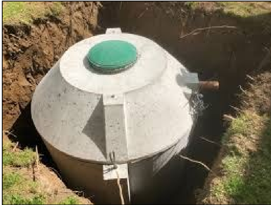
Plate 4-13: Typical rainwater harvesting tank used on wind farms
