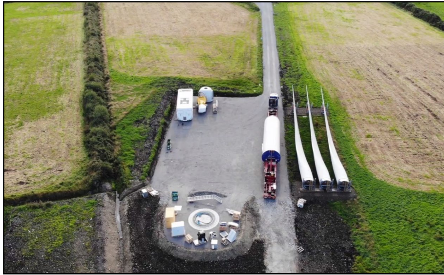
Plate 4-2: Example of a typical Wind farm finished wind turbine hardstand area
