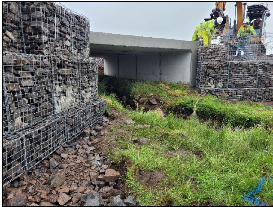
Plate 4-17: Example of a clear span pre-cast concrete box culvert over a watercourse/drain
