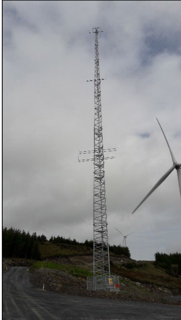
Plate 4-6: Example of a typical Meteorological Mast on a wind farm
