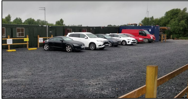
Plate 4-7: Example of a typical temporary construction compound on a wind farm
