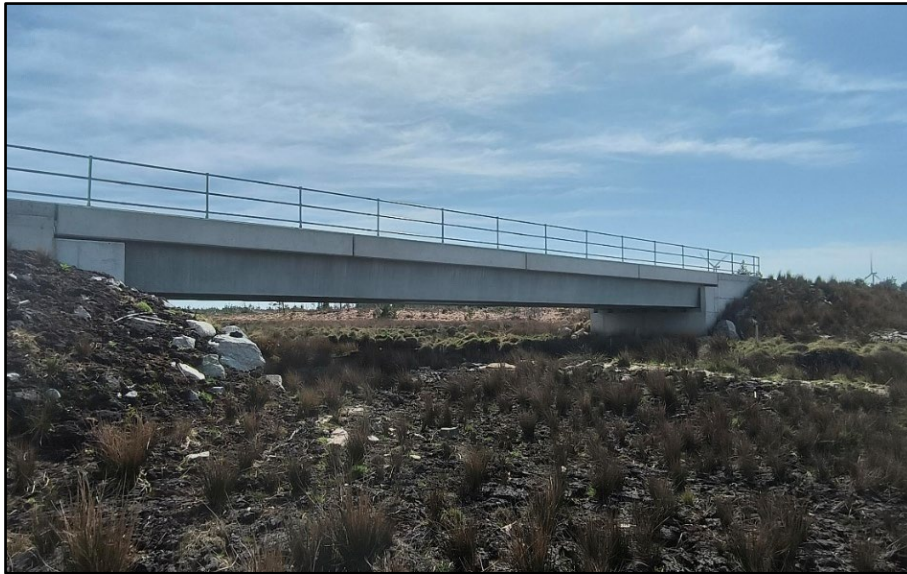
Plate 4-16: Typical clear span crossing used on wind farms
