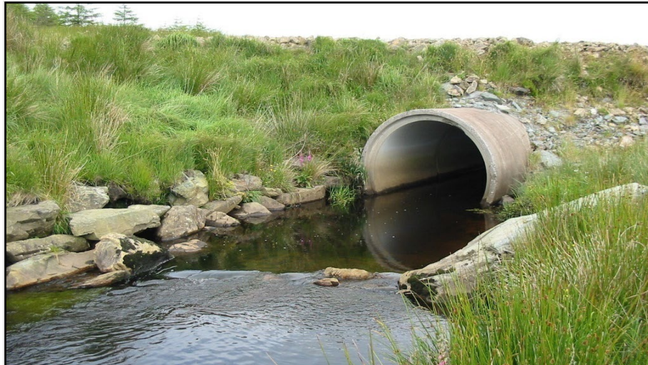
Plate 4-18: Example of a concrete pipe culvert for a watercourse/drain crossing
